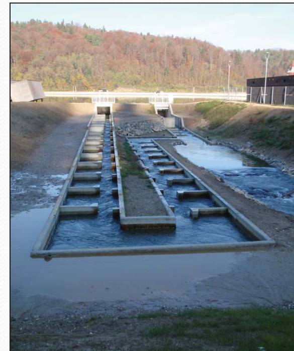
Upper intake reach with vertical slots
