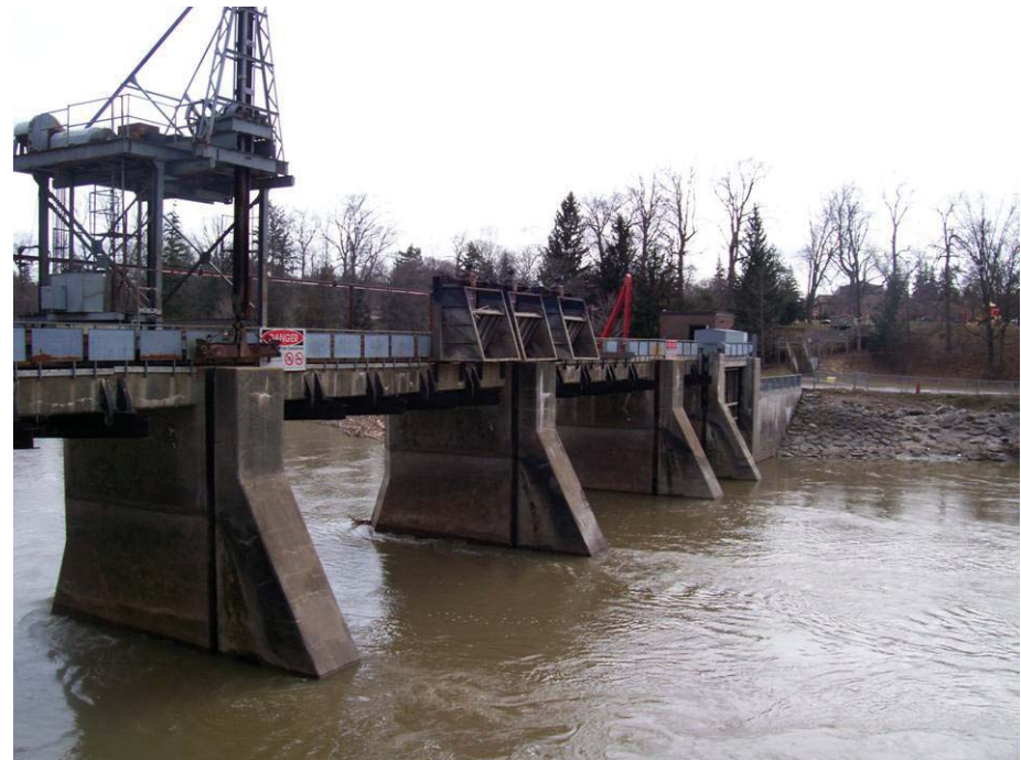
Springbank Dam, Upper Thames, London, ON
